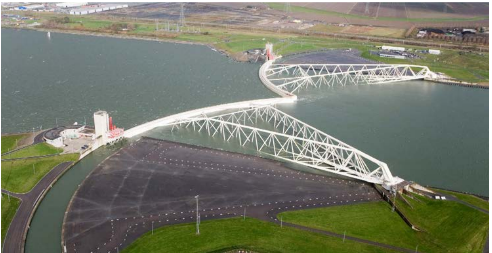
Reference for Alternative 1: Maeslantkering, The Netherlands Source: Rijkswaterstaat
