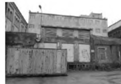
A11 Old power plant
