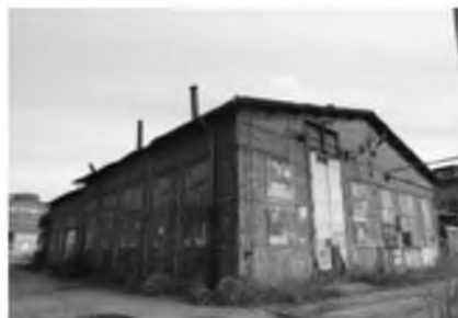
40 A Equipment production Hall
