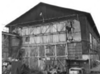
41 A Equipment fabrication Hall
