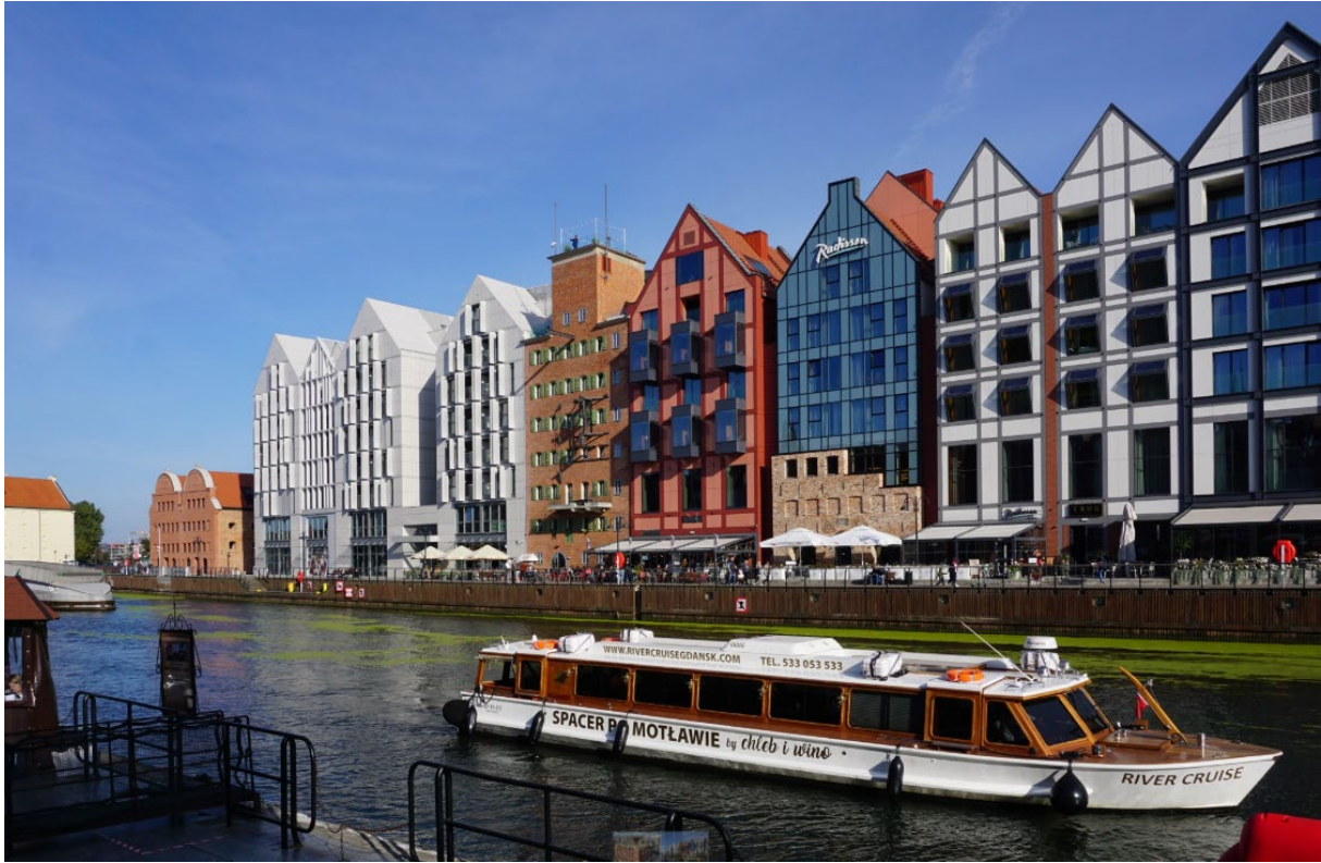
Recently rebuilt northern tip of the Granary Island
