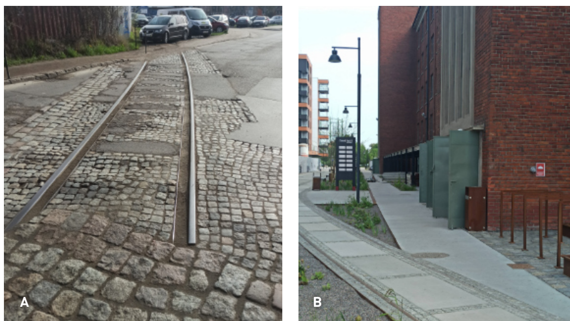
Fig. 58 A-B. challenge for the area is to reconcile universal design with heritage protection in the form of remnants of historical pavements, including railway and crane tracks (old track beds); on the left, pavement remnants and old track bed in Narzędziowców Street designated for removal; on the right, the reconstructed route of the old track bed of branch line 105 of the Gdańsk Shipyard around the Montownia food hall. Source: Piotr Smolnicki, April 2024, Autumn 2025.
