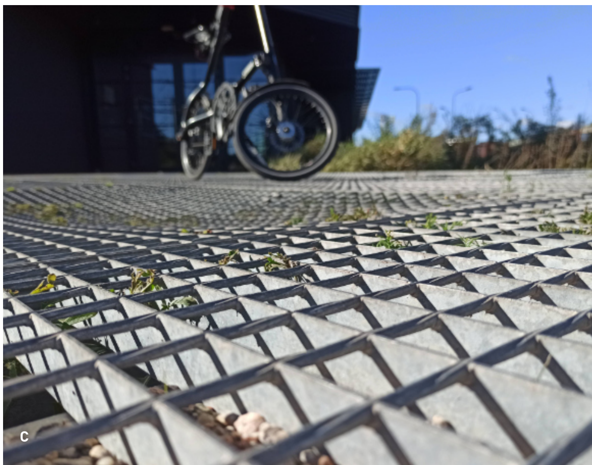
Fig. 43 A-C. Example of the type of bridge truss used in the Young City – corner of ks. Jerzego Popiełuszki and Rybaki Górne streets. Source: Piotr. Smolnicki, A, B – autumn 2025, C – October 2024.
