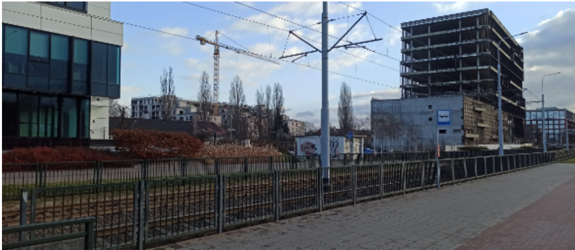
Fig. 56. Unfinished office investment at 183 Marynarki Polskiej Street as a mental barrier: visually unattractive, not welcoming due to a lack of services, and creating a sense of insecurity. Source: Piotr Smolnicki, Autumn 2025.
