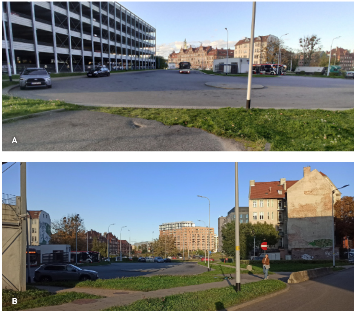
Fig. 60 A-B. Area barriers in the form of development unsuitable for a central urban function: a multi-storey parking structure with a bus depot and blind walls of historic tenement houses. Source: Piotr Smolnicki, Autumn 2025.
