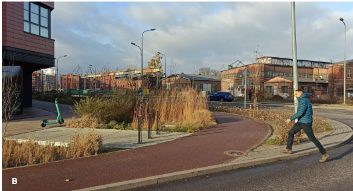
Fig. 50 A-B. Lack and insufficient number of pedestrian crossings on Rybaki Górne Street. Source: Piotr Smolnicki, Autumn 2025.
